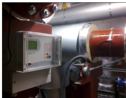
KATflow 150 for heat quantity measurement application using PT100 sensors
